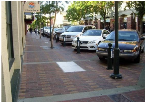
BRICK PAVERS IN URBAN PLAZA AREA
