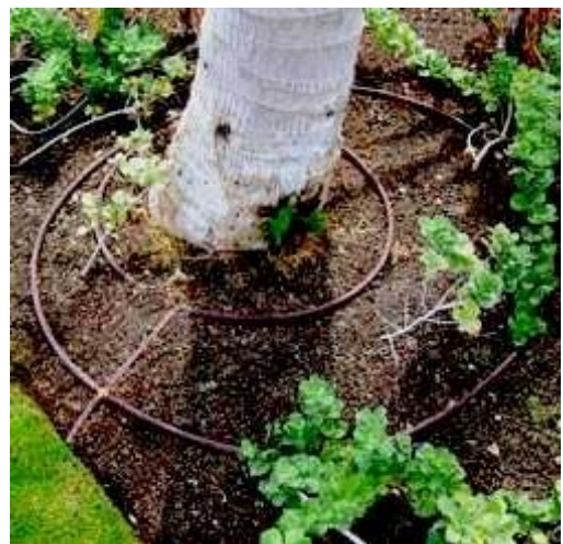
STREET TREE DRIP IRRIGATION
